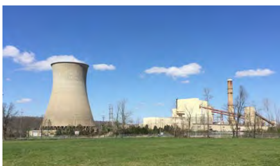
Figure 1: William H. Zimmer Generating Station
