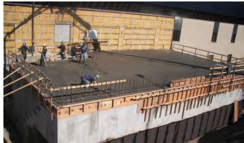
Figure 5: October 2012: concrete casting.
